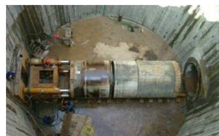
▲ Pipeline pushing project in city highway construction.
