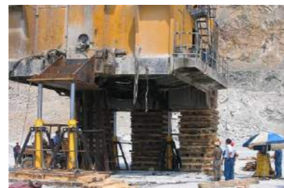
▲ Synchronous lifting and maintenance of large mining machinery.
