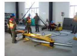
▲ Bending of cable pipelines in nuclear power plants.
