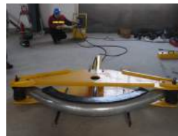
▲ Bending of cable pipelines in nuclear power plants.
