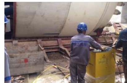
▲ Synchronous pushing in position of shield machine.
