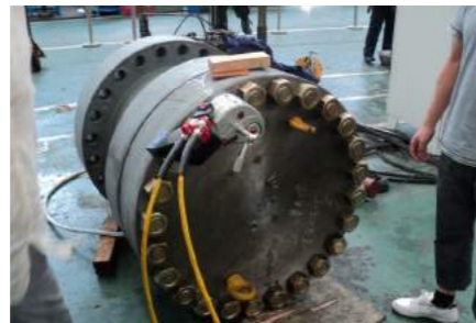
▲ Bolt tightening of high pressure pipe flange in steel plant.
