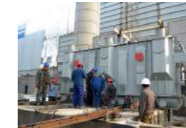
▲ Pushing-moving in position of transformer in thermal power plant.
