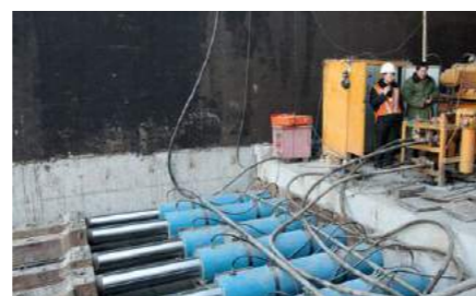
▲ Box culvert pushing project in highway construction.
