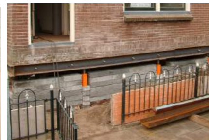
▲ Synchronous lifting and moving of building.
