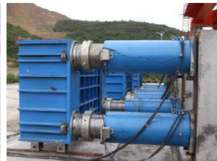
▲ Synchronous pushing of prefabricated beam in high speed rail construction.
