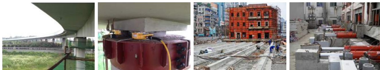
▲ Synchronous lifting and replacement of highway bridge rubber bearings.
