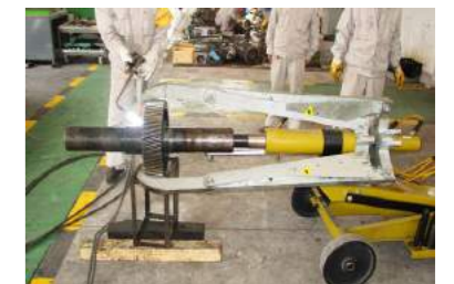
▲ Gear disassembly for equipment maintenance in thermal power plant.
