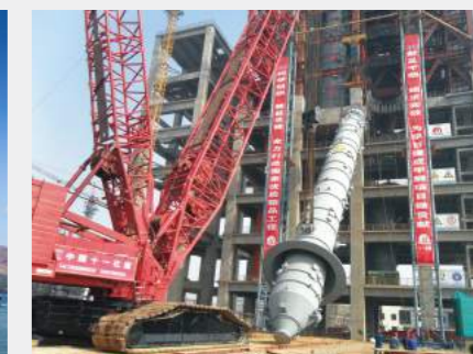
▲ Synchronous lifting and installation of pressure vessel installation in refinery.
