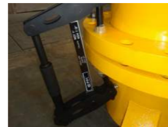
▲ Pipe flange adjustment in chemical plant.
