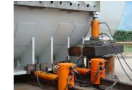
▲ Pushing-moving and installation of generating equipment in thermal power plant.
