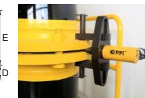
▲ Packing replacement of high pressure pipe flange in thermal power plant.
