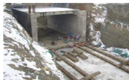
▲ Box culvert pushing project in highway construction.
