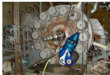
▲ Bolt disassembly of high pressure water pump in thermal power plant.
