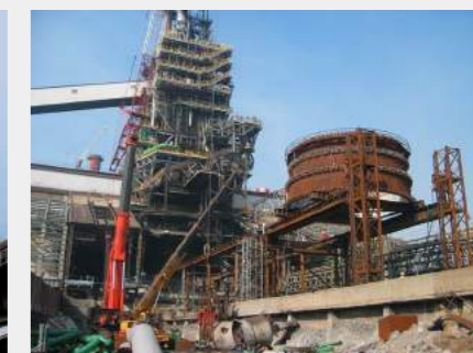
▲ Synchronous lifting of blast furnace in steel plant.
