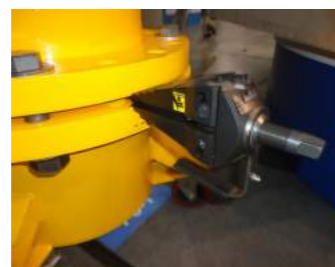
▲ Packing replacement of high pressure pipe flange in oil refinery.
