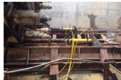
▲ Synchronous pushing in position of shield machine.
