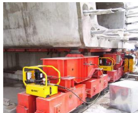
▲ Synchronous lifting and transferring of high-speed rail box girder.
