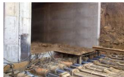
▲ Synchronous pushing of box culvert in high speed railway construction.
