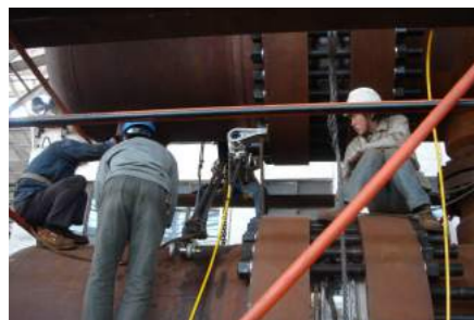
▲ Bolt tightening of pressure vessel in oil refinery.
