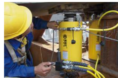
▲ Synchronous lifting and installation of steel structure.
