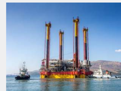
▲ Synchronous lifting and installation of offshore oil drilling platform.
