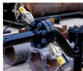
▲ separate pipeline flange to replace seals in refinery.
