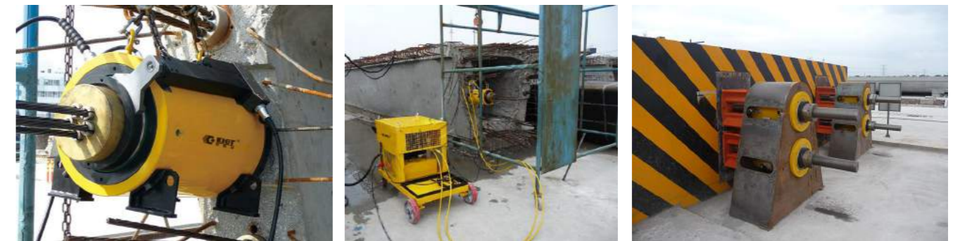
▲ Prestressed tensioning of high-speed rail box girder.
