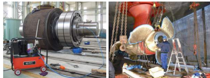
▲ Bearing installation of grinding roller maintenance ▲ Propeller installation in shipyard in cement mill.
