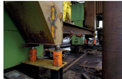
▲ Synchronous lifting of hull in shipyard.
