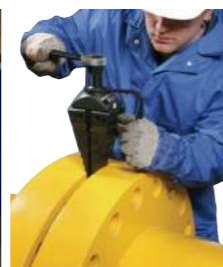
▲ Seals replacement of oil pipe flange.
