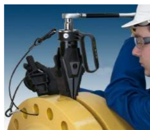
▲ Seals replacement of high pressure pipe flange in paper mill.
