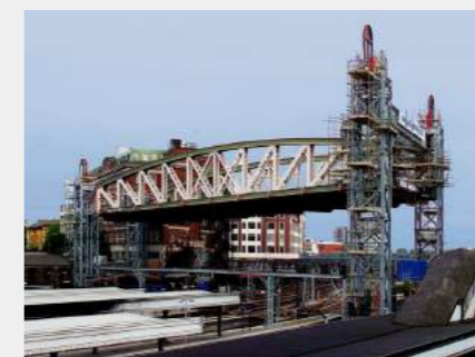
▲ Synchronous lifting and installation of highway corridor.
