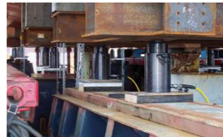
▲ Synchronous lifting and installation of large steel structure bridge.
