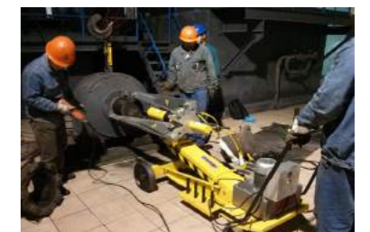
▲ Large single pulley disassembly in thermal power plant.
