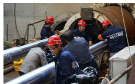
▲ Pipeline pushing project in high speed railway construction.
