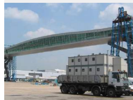
▲ Synchronous lifting and installation of air corridor.
