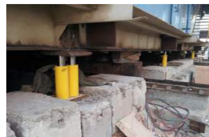
▲ Synchronous lifting and maintenance of large equipment.
