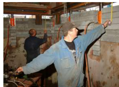
▲ Synchronous lifting and moving of building.
