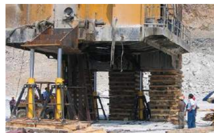
▲ Synchronous lifting and maintenance of large mining machinery.
