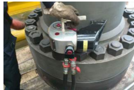
▲ Bolt pre-tightening of high pressure pipe flange in Chemical plant.
