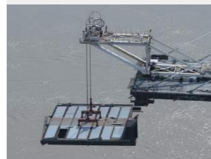
▲ Synchronous lifting and installation of steel structure bridge.
