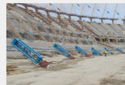
▲ Synchronous lifting and installation of stadium dome.
