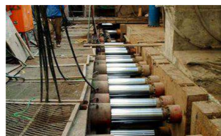
▲ Box culvert pushing project in highway construction.
