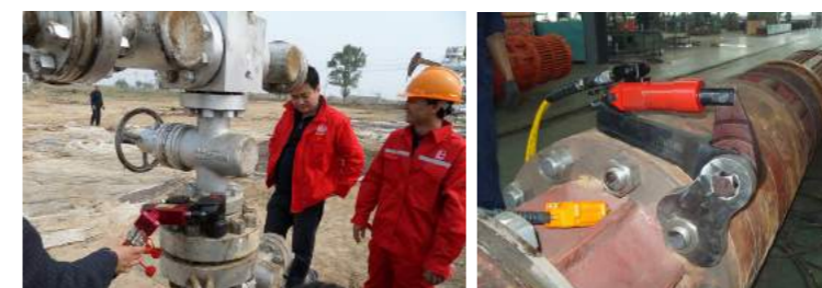
▲ Bolt tightening of pipeline flange in West-East natural gas transmission project.
