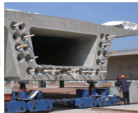
▲ Synchronous pushing of prefabricated beam in high speed rail construction.
