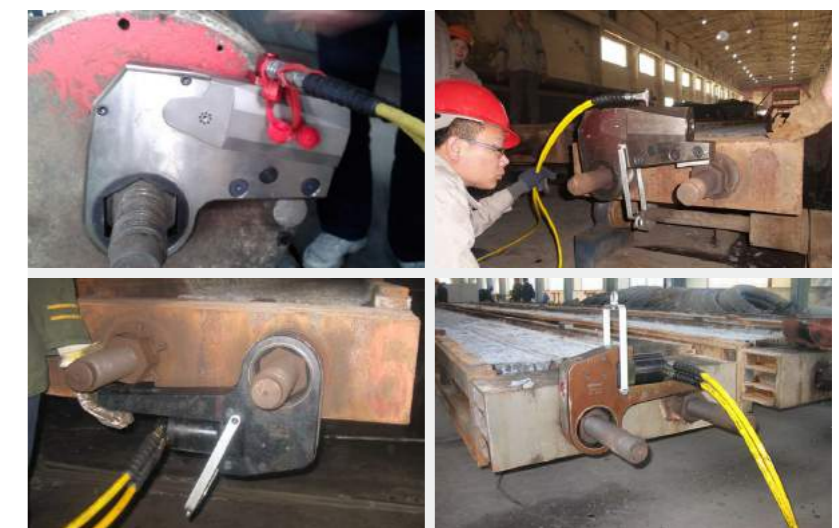
▲ Bolt tightening in sleeper factory
