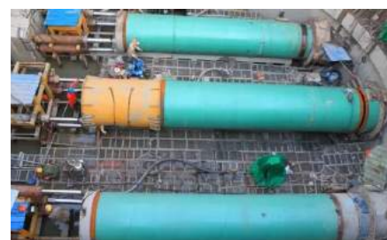
▲ Pipeline pushing project in railway construction.
