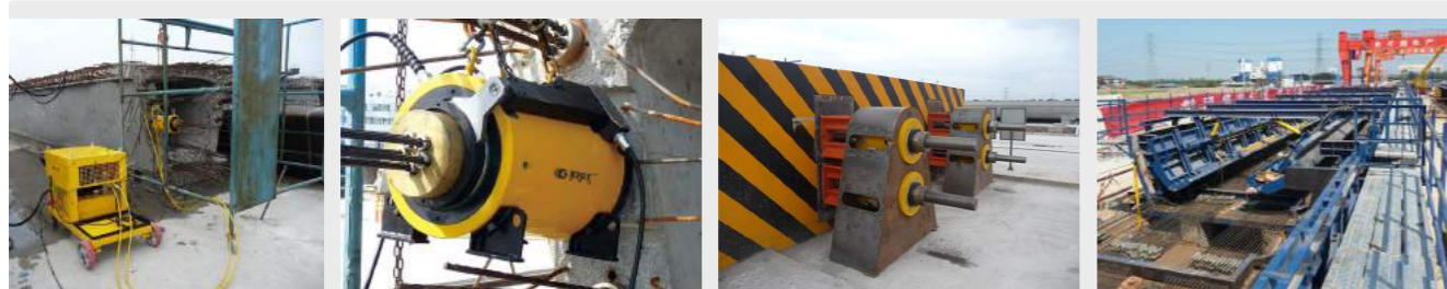
▲ Prestressed tensioning of high-speed rail box girder.
