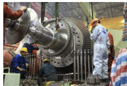
▲ Bolt disassembly of turbine in thermal power plant.
