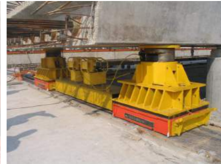
▲ Long term supporting for high-speed rail box girder prefabricating.
