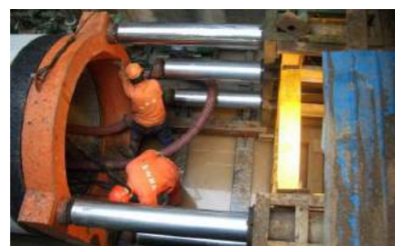
▲ Pipeline pushing project in expressway construction.
