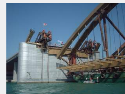
▲ Synchronous lifting and installation of large bridge structure.
