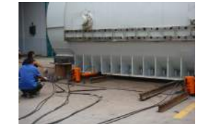
▲ Pushing-moving in position of generating equipment in thermal power plant.
