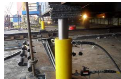
▲ Synchronous lifting and docking of shipbuilding.
