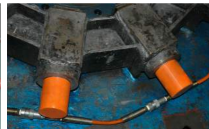
▲ Synchronous locking of cable of cable-stayed bridge in bridge girder construction.
