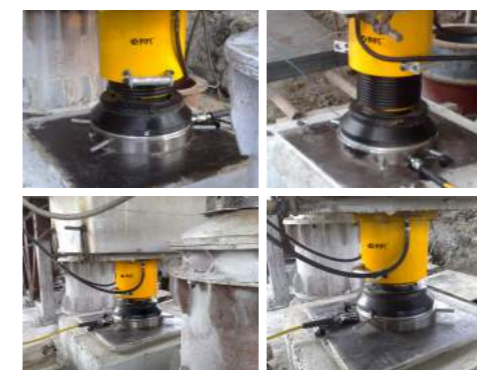
▲ Synchronous lifting for increase the clearance of large bridge.
