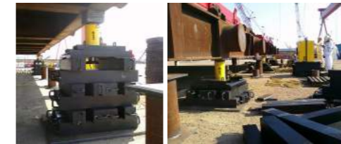
▲ Welding and lifting for vessel body
